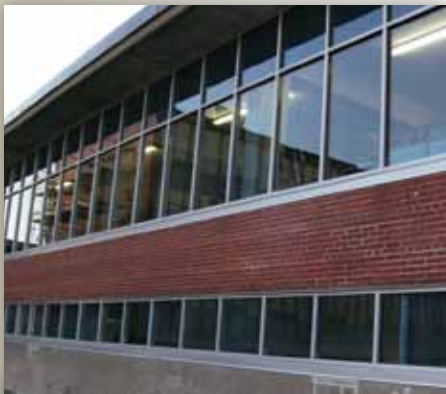
A high-efficiency tinted window system dramatically changed the look of the high school's exterior.
