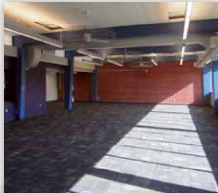
The high school's interior spaces were redesigned to feel more spacious and incorporate natural light.
