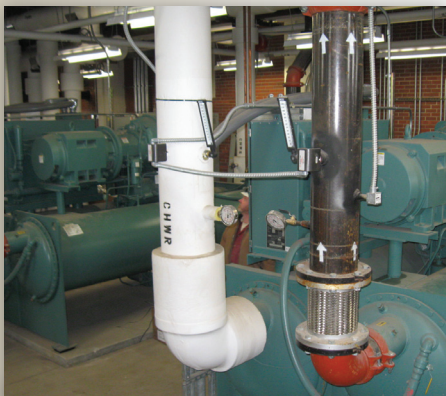
Phase 2 of the project included a $2.4 million mechanical equipment upgrade and a new Physical Plant.
