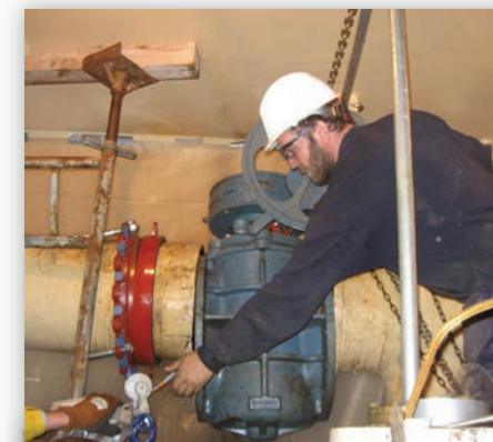
Workers install one of the isolation valves; each weighs approximately 1,000 lbs.
